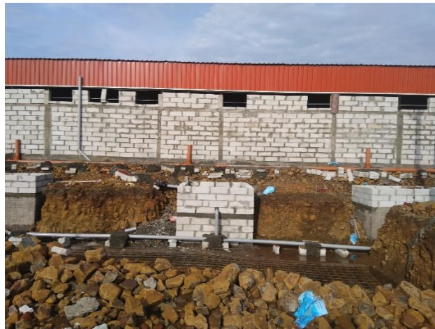
Bio-chamber structures being built behind the dormitory
