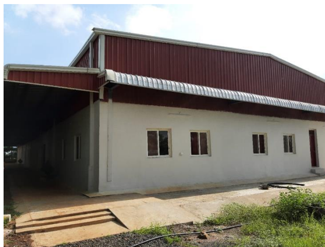
Mokshadham Dormitory front side
