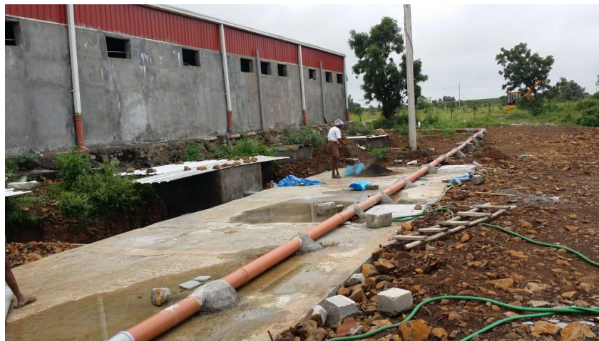
Settling tank completed and Aquatron® units protected with metal sheets.
