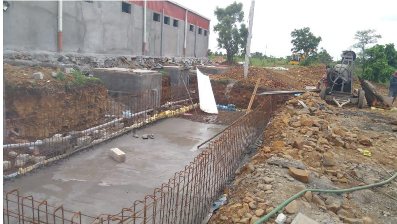
Settling tank being built. Bio-chambers visible at the back.
