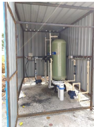
Simple water treatment plant at Quantum Life University
